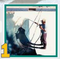
Clean Substrate. Remove loose, delaminated plaster and contaminants.
